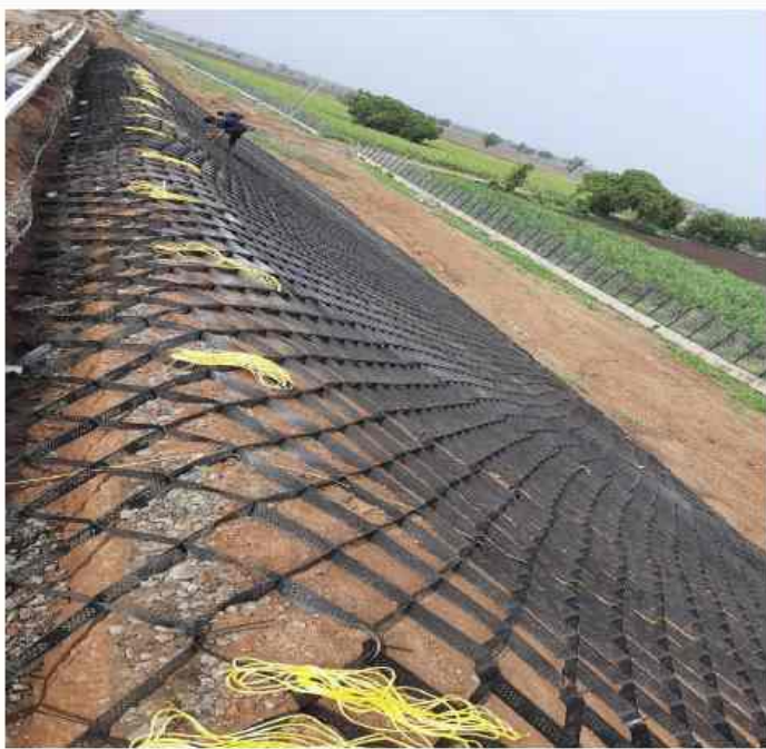
CH 303+850 Geo cell laying work in progress
