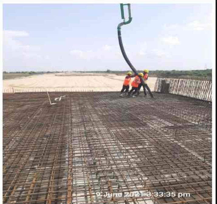
CH 297+472 MNB Deck slab concrete pouring work in progress
